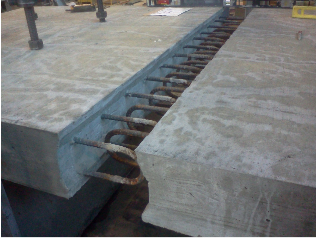
Figure 3.11: Specimens set in place to form the joint prior to sandblasting
