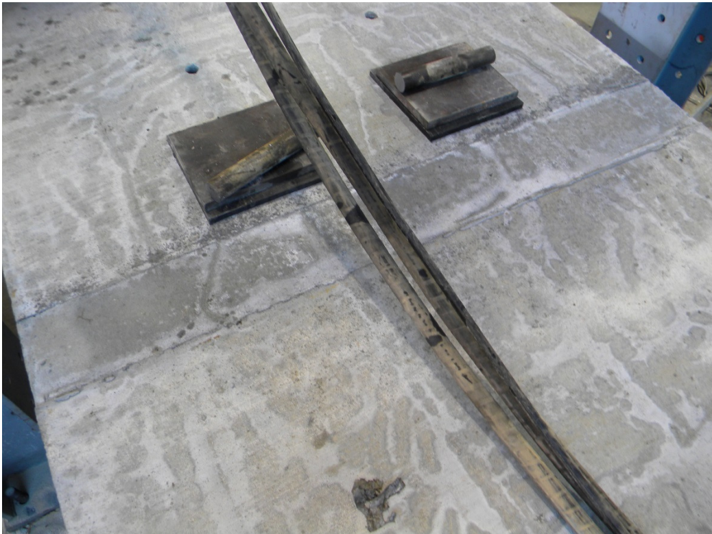
Figure 3.14: Joint following closure pour
