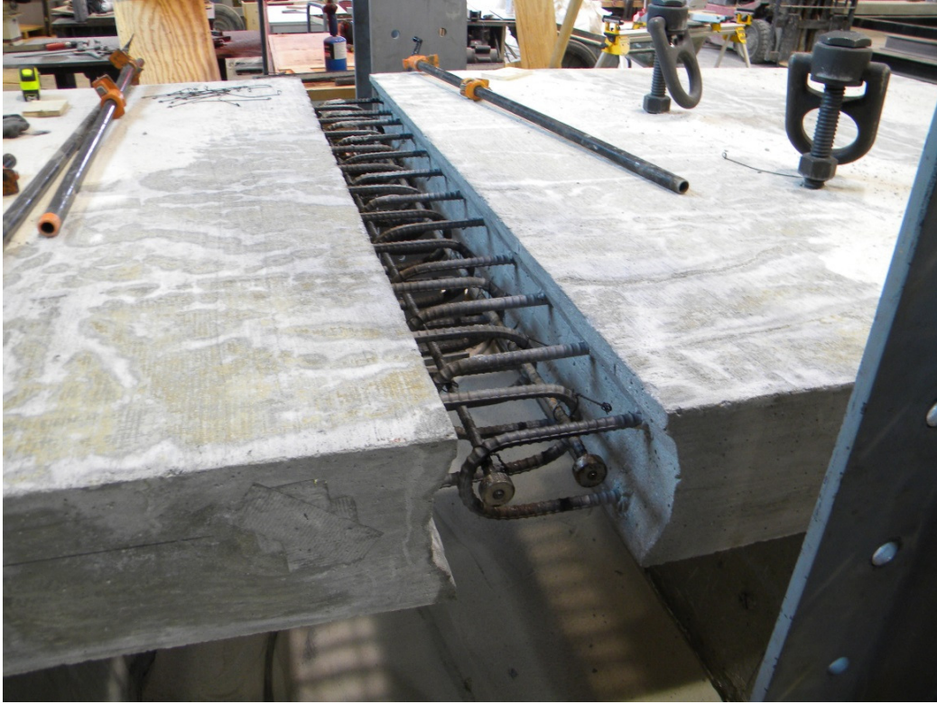
Figure 3.13: View of completed joint prior to pour
