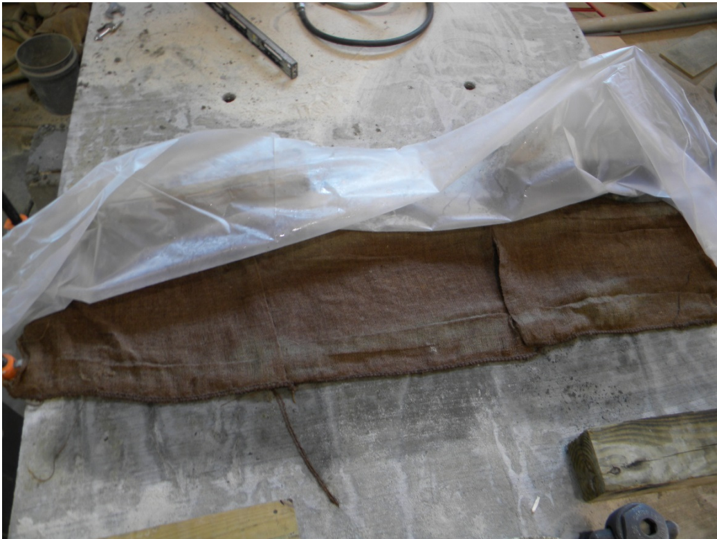
Figure 3.16: Burlap and plastic used for curing joint
