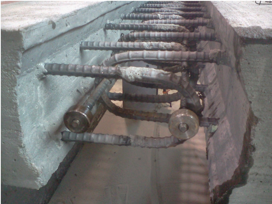
Figure 3.12: Joint formed with #4 headed bars in position following sandblasting
